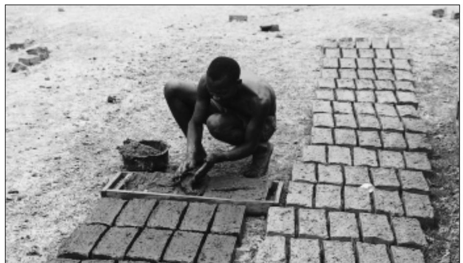
Fig. 4: Correct drying process: green bricks dry slowly in the open in cloudy weather, thus developing no cracks and deformation
