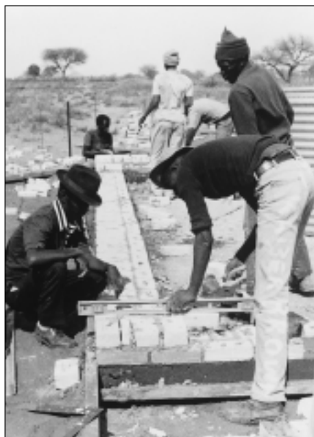
Fig 2: Building with burnt bricks in Zimbabwe.
