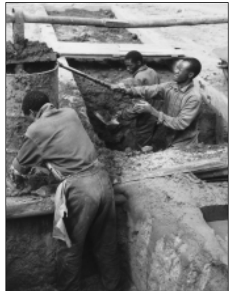
Fig 4: Filling a pugmill with clay.
