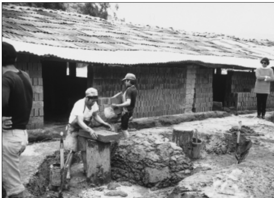
Fig 3: Demoulding clay bricks by hand in Cajamarca, Peru.
